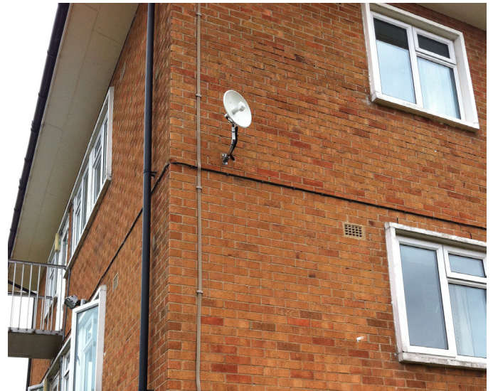
NanoBeamM5 CPE Mounted to the Side of the Barracks
