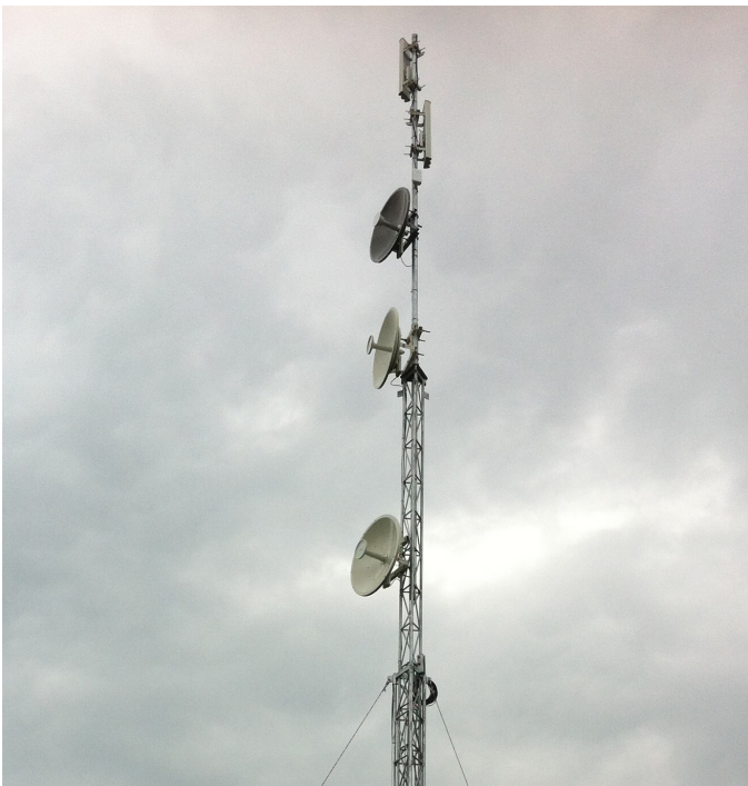
RocketM5 Access Points Attached to RocketDishes and Sector Antennas
